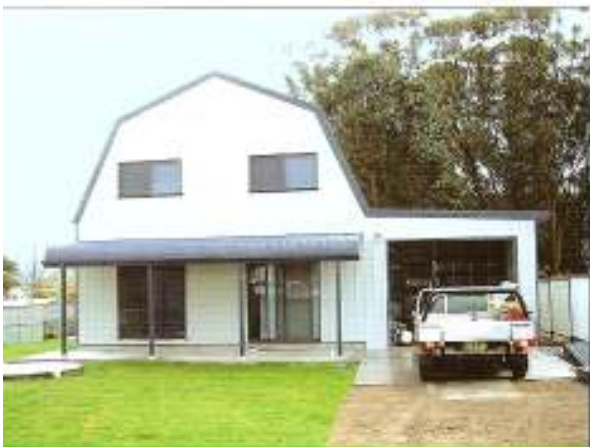
Quaker Barn with closed-in lean-to
