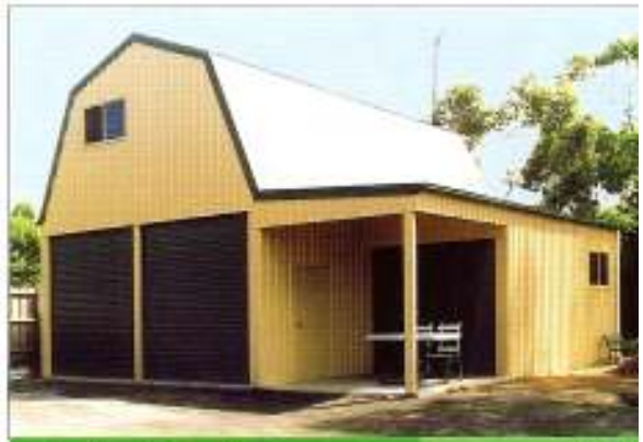
Quaker Barn with partially closed-in lean-to
