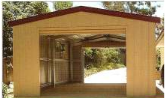
Single Garage with roller doors front & rear
